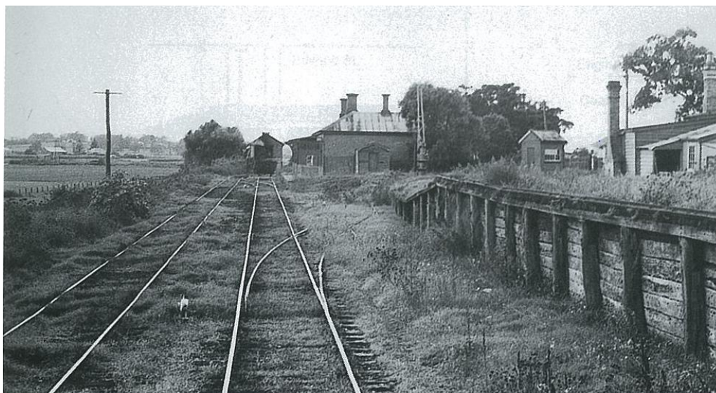
Figure 19. The terminus on 12 March 1953. The timber-faced loading bank, next to which runs the barely-visible goods siding, is at right; behind it is the weighbridge associated with the trucking yard; the 5-ton capacity manually-operated jib crane; the former passenger station; and the engine shed. The goods shed has already been demolished. The cottage at extreme right, perhaps former commercial premises, known as 36 Swan Street, still stands. Late C.C. Singleton
